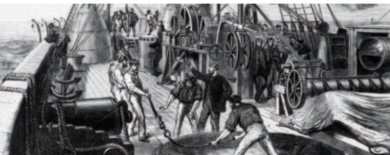
Laying the Atlantic Telegraph Cable from the steamship 'Great Eastern', from the Illustrated London News, September 2, 1865.
