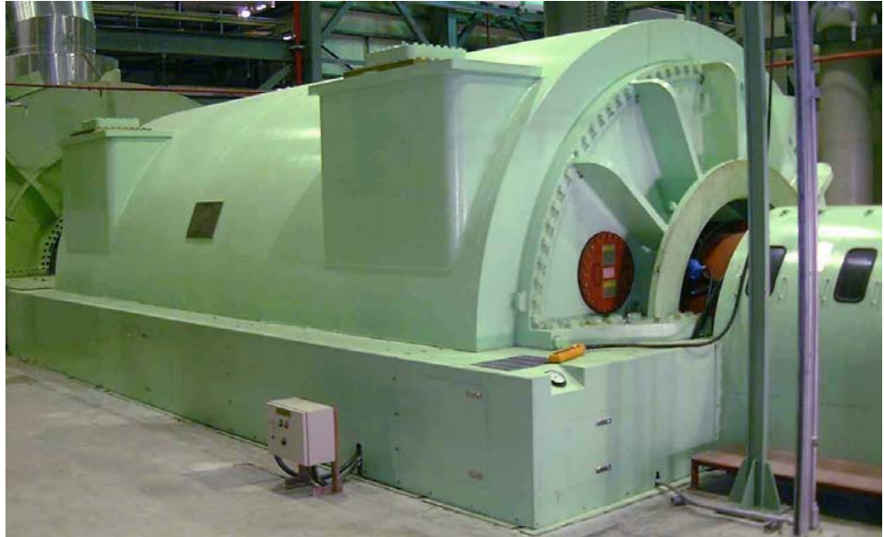
Figure 8: Hydrogen-Cooled Generator
