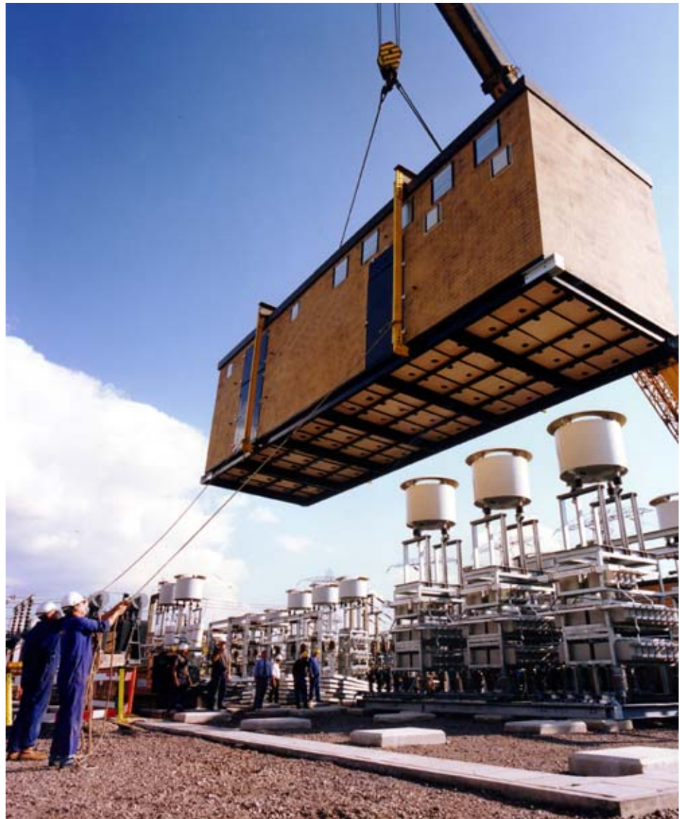
Figure 4: Installation of Mobile SVC
