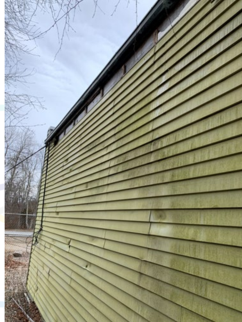
Canonicus Switchyard Building Exterior
