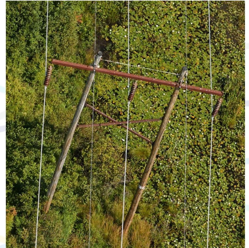
Typical Structure Condition on S-171N & T-172N Str 14
