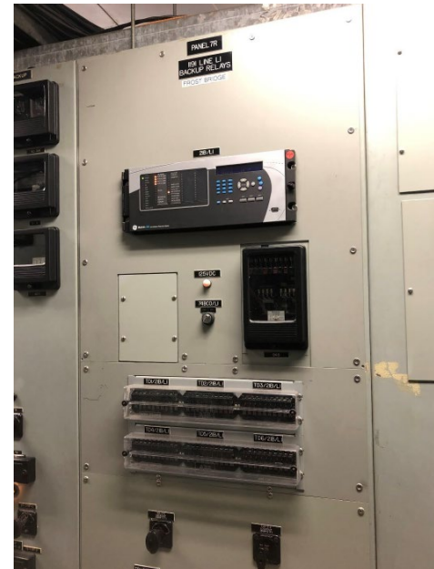
Campville - GE 115 kV Line 1191 Relay
