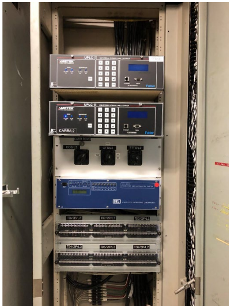
Campville - SEL 115 kV Line 1900 Relay
