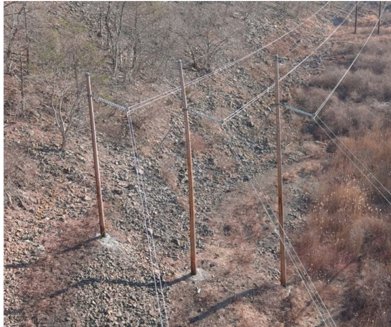
Line 3041 - Structure 9564 Leaning Poles & Washout Concerns
