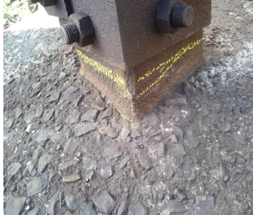
Line 3041 - Structure 9551 Section Loss
