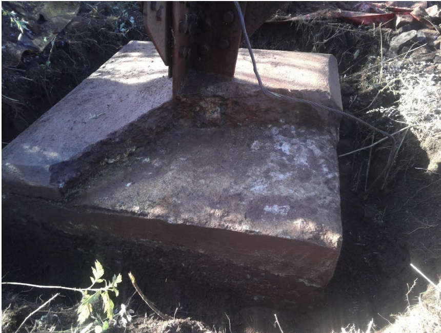
Line 3754 - Structure 8717 Deteriorated concrete, steel foot of structure leg exposed with rust and corrosion
