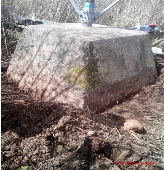
Line 3041 - Structure 9500 Foundation Deterioration
