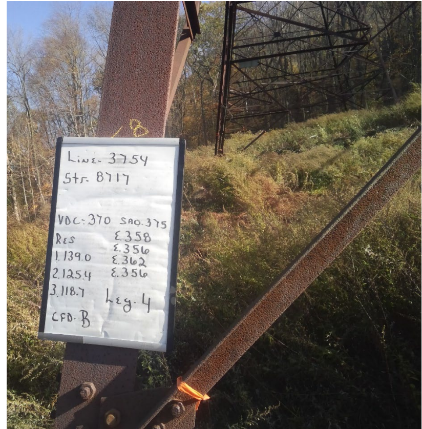
Line 3754 – Structure 8717 Rust and pitting of galvanized steel structures
