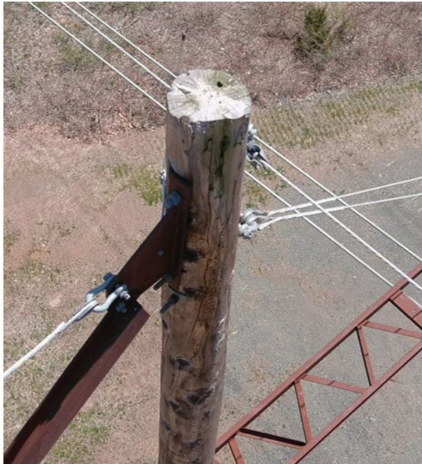
Line 3041 - Structure 30020 Splitting Pole Top
