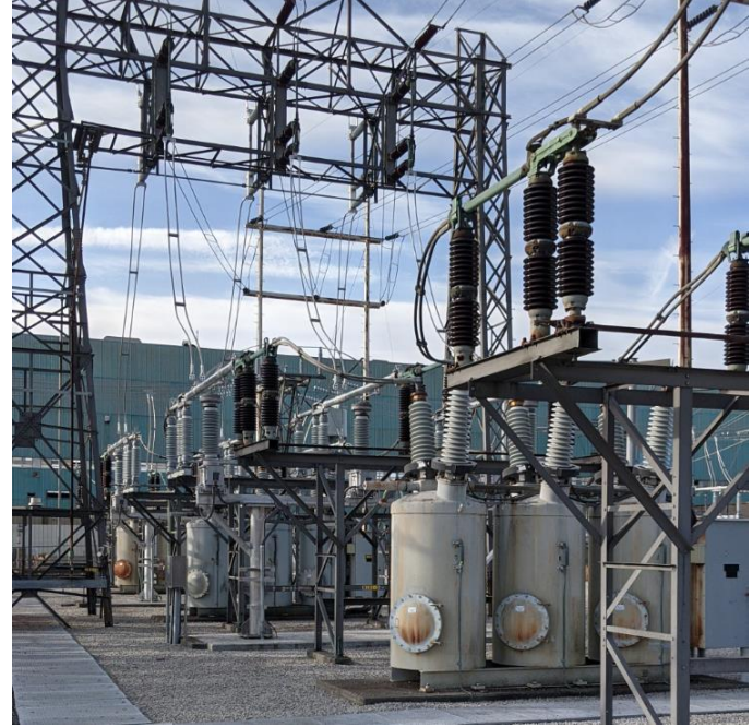
115kV BZO Oil Circuit Breakers
