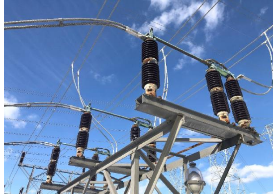
115kV group operated disconnects
