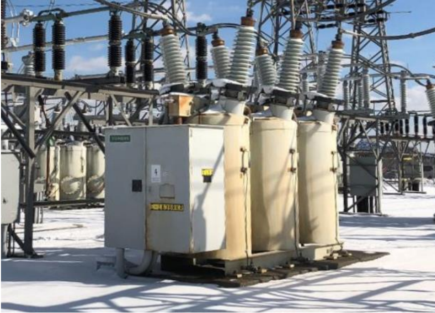
115kV BZO Oil Circuit Breakers
