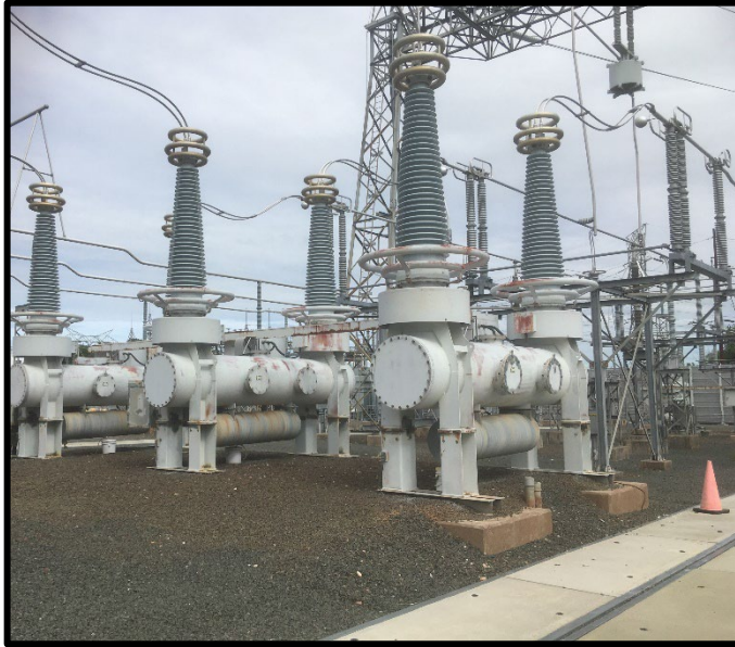
345 kV breaker at Manchester Substation
