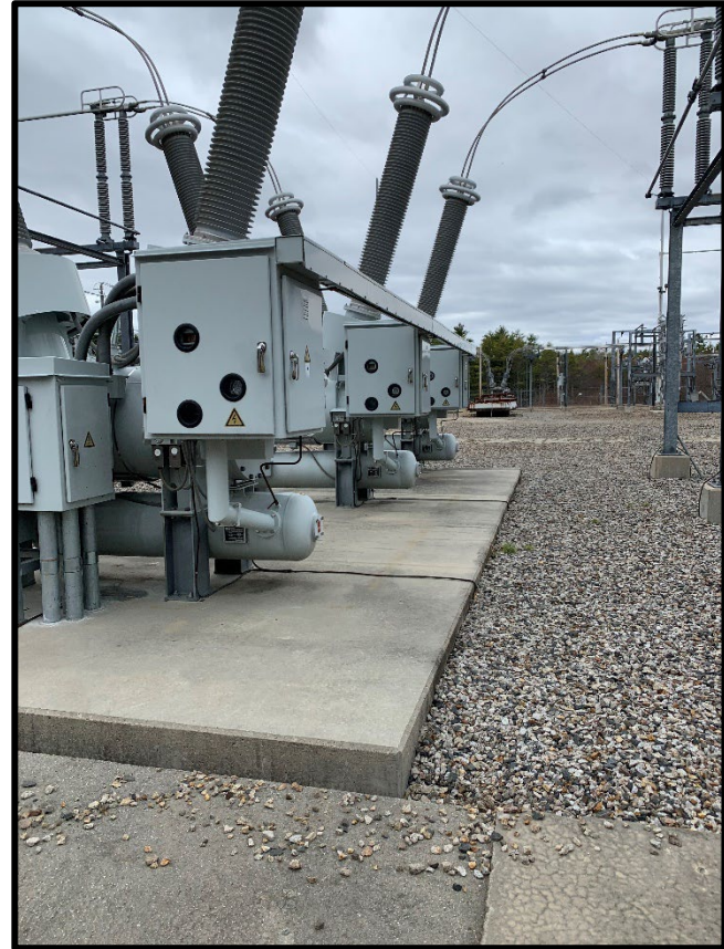
345 kV breaker at Amherst Substation
