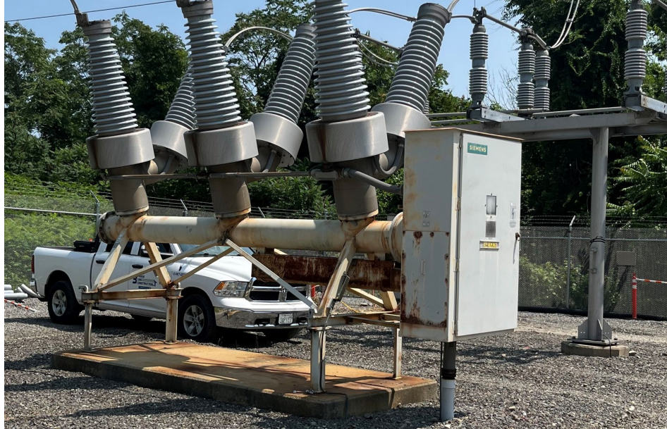
115 kV Gas Circuit Breaker #141
