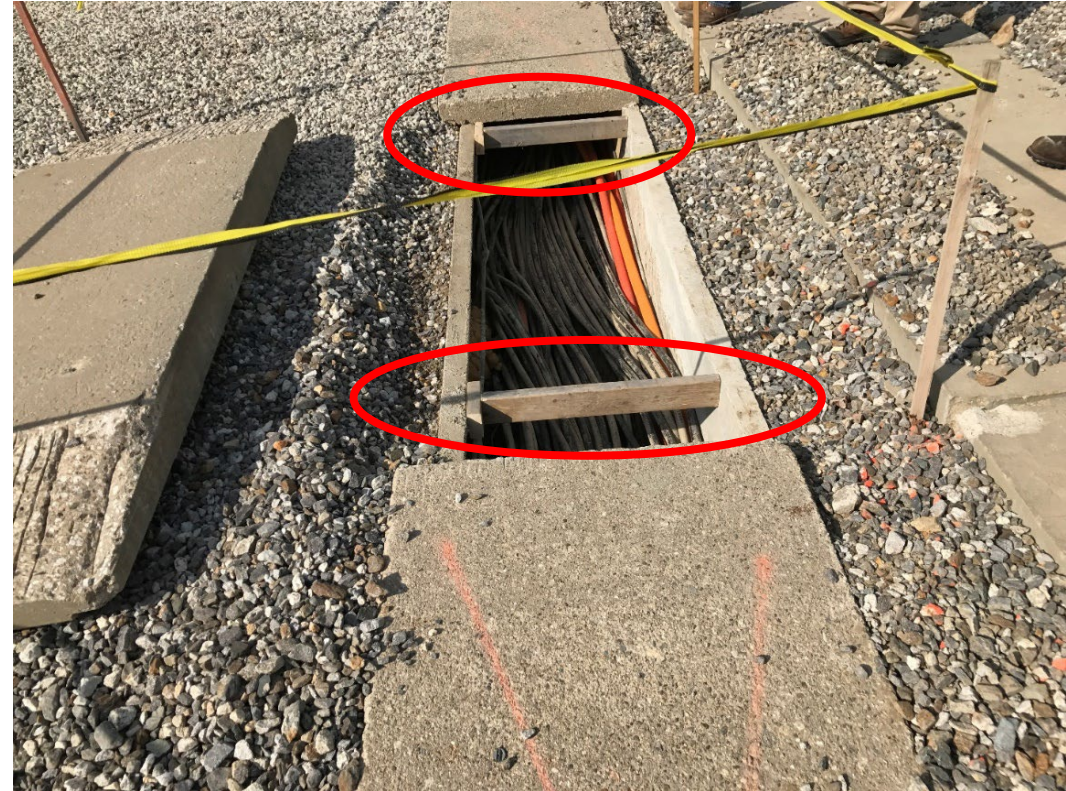
Left Sidewall Collapsing Into Trench and Braced with 2'x4's
