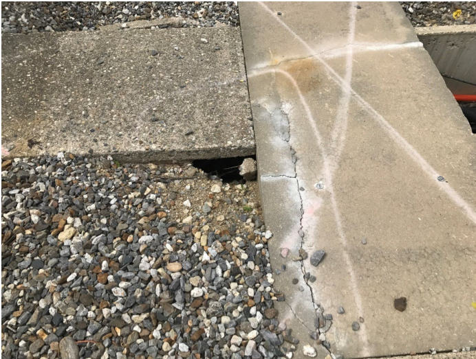
Cracking of Concrete Cover
