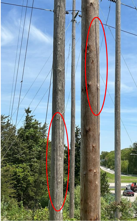
S-171S Structure 263 - Back Pole Cracks
