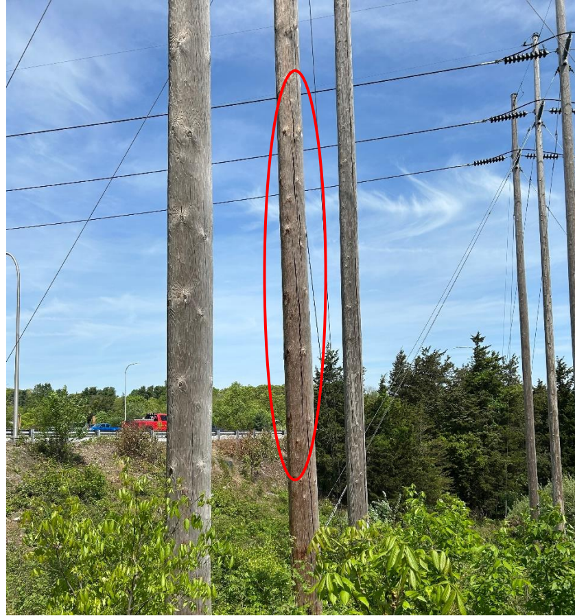
S-171S Structure 263 - Front Pole Cracks
