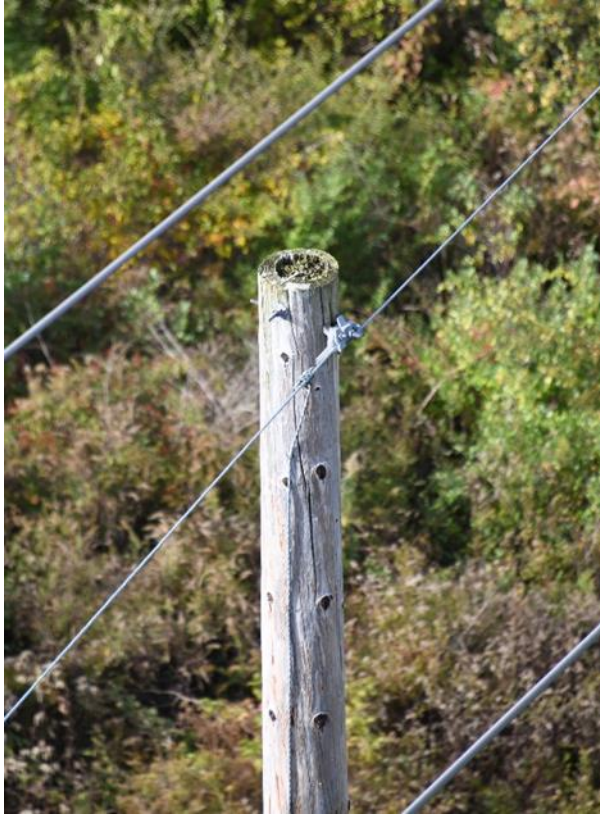
S-171S Structure 224 Pole Top Rot
