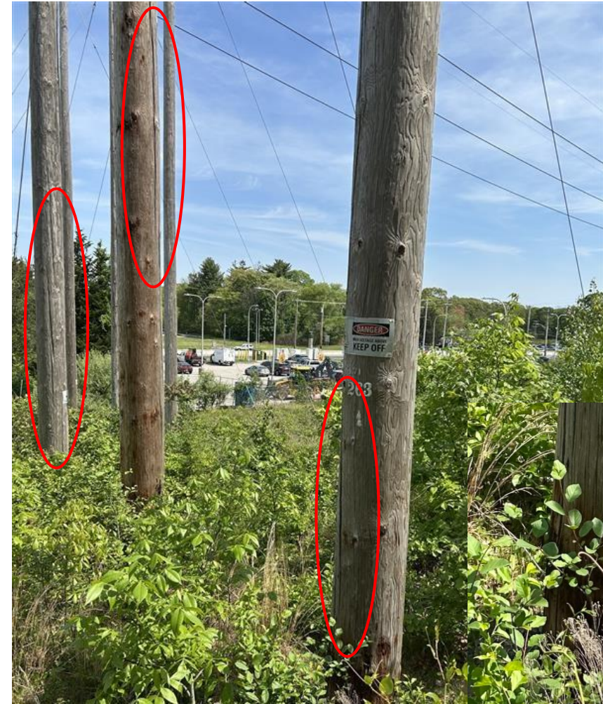
S171S Structure 263 Pole Cracks and Pole Base Deterioration
