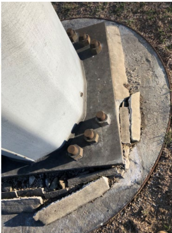
Foundation Damage on E-183W Str 180
