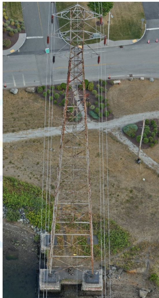
Severe Paint Chipping and Deterioration on E-183W Str 204
