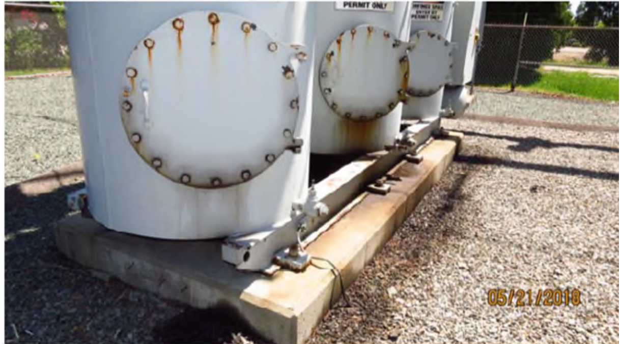
Signs of oil leak on the B-phase of the 9801 breaker
