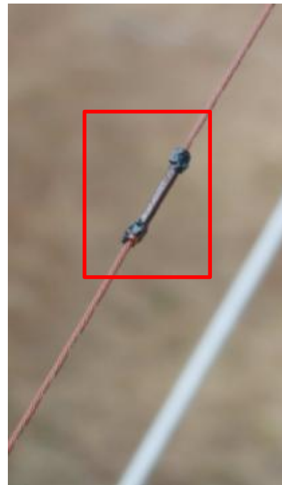
Frequent splices in shieldwire across entire circuit
