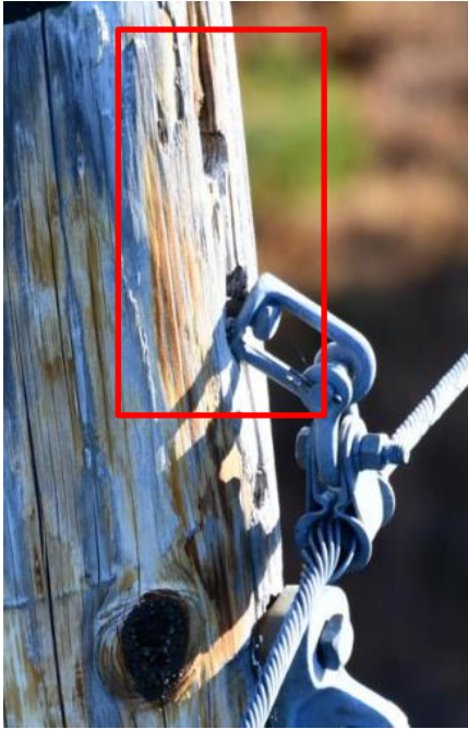
E-205E Str. 868 Installed 2009
