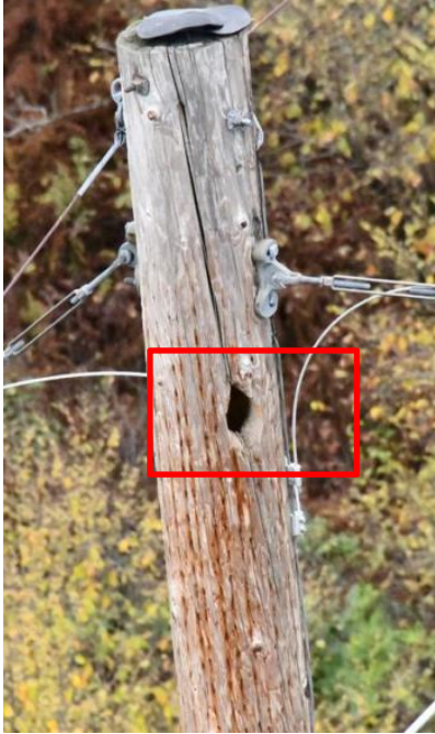
E-205E Str. 701 Installed 1995
