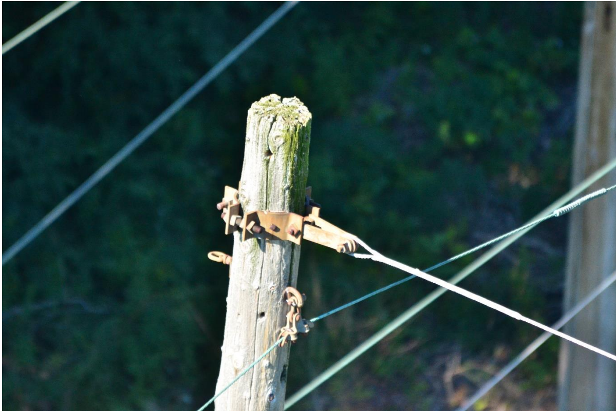
Structure 3657 – Pole top split, woodpecker damage
