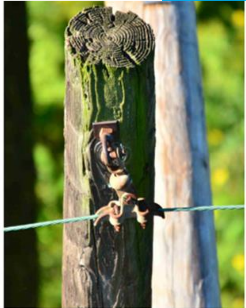
St. # 4567 Woodpecker damage and rotten pole tops
