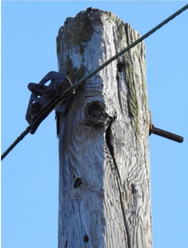
St. # 4575 Splitting and rotten pole tops
