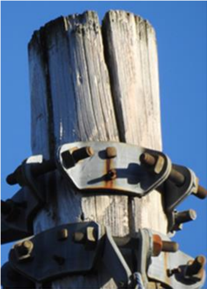
St. # 3657.5. Splitting and rotten pole tops
