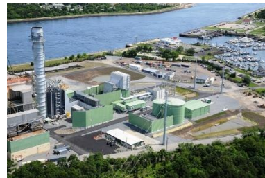
NRG Canal 3 Sandwich, MA 333 MWs Online June 2019
