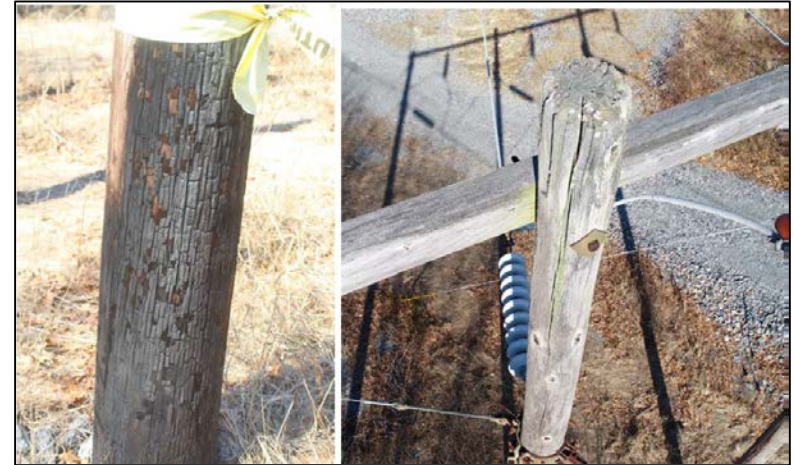
Structure #8343 – Split pole tops, woodpecker damage, cracks, burnt at base
