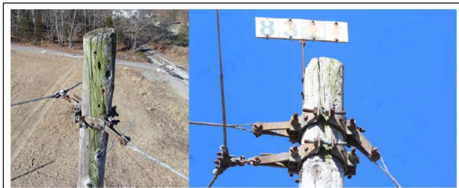
Structure #8345 – Split pole tops, woodpecker damage
