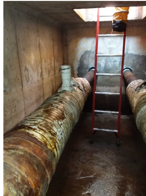
Typical Pipe Degradation – Line 282-520
