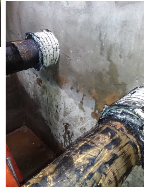
Typical Pipe Degradation – Line 282-520
