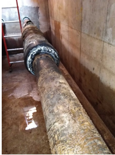
Typical Pipe Degradation – Line 282-521
